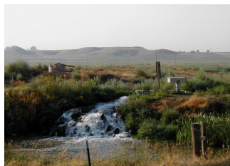
WR Jones Ditch Augmentation Structure
