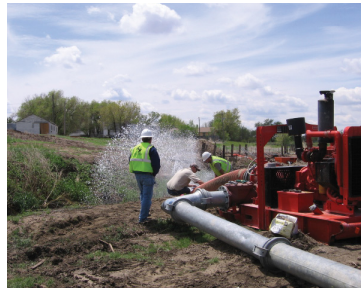
Pumping water into Nissen Recharge Pond
