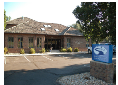
Central's office at 3209 W 28th Street, Greeley, Colorado
